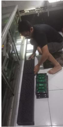
Figure 11. Installation of LED Panels
