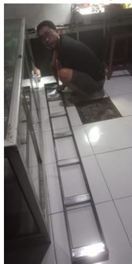
Figure 10. Installation of Elbows and Keys
